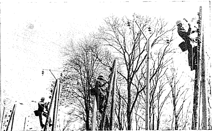
Above: Some of the French linesmen on a re-training course at the overhead line section of the School.
