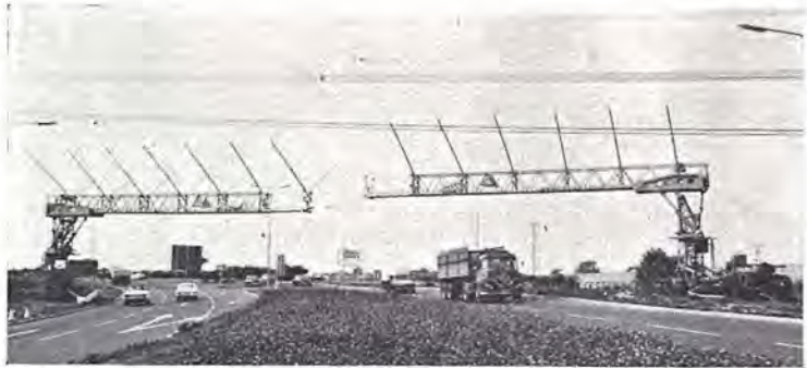
The CEGB 'Sky Cradle' stretched across the dual carriageway at Eiton.
